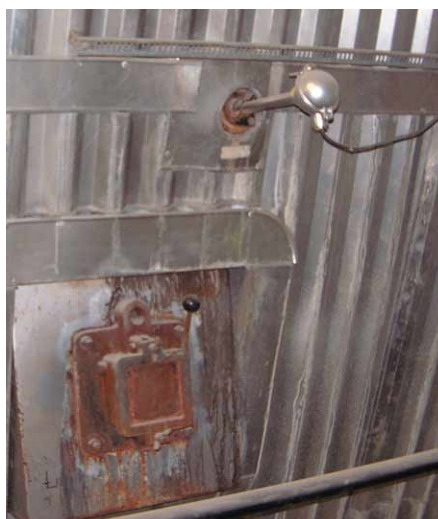
Sensor with "metal-ceramic" sheathing measuring the temperature of the firebox, positioned next to an inspection hole. Incineration plant in Le Mans.
