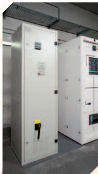
Fig. 4 – Recording of the power profile with the capacitor bank
